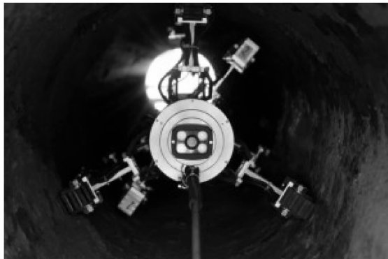
图 5 爬行机器人检测实物图 Figure 5 Picture of crawling robot detection
